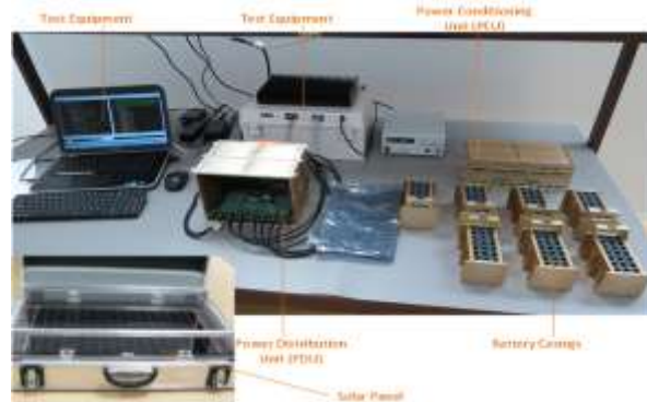
Power Distribution Unit
